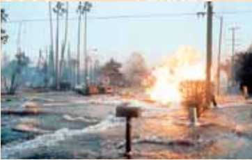
Gas escaping from a broken pipe burns as water from a ruptured main floods a Los Angeles street after an earthquake Source: L. Ignelzi.
